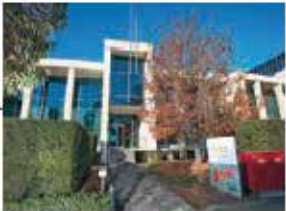
PORT MELBOURNE 684 Lorimer Street Port Melbourne VIC 3207 Australia
